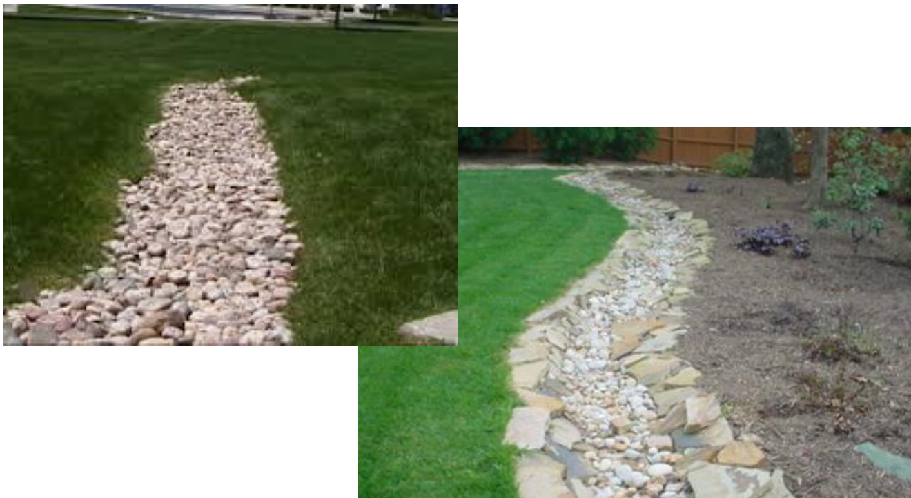
Figure 12: Infiltrating gravel drains
