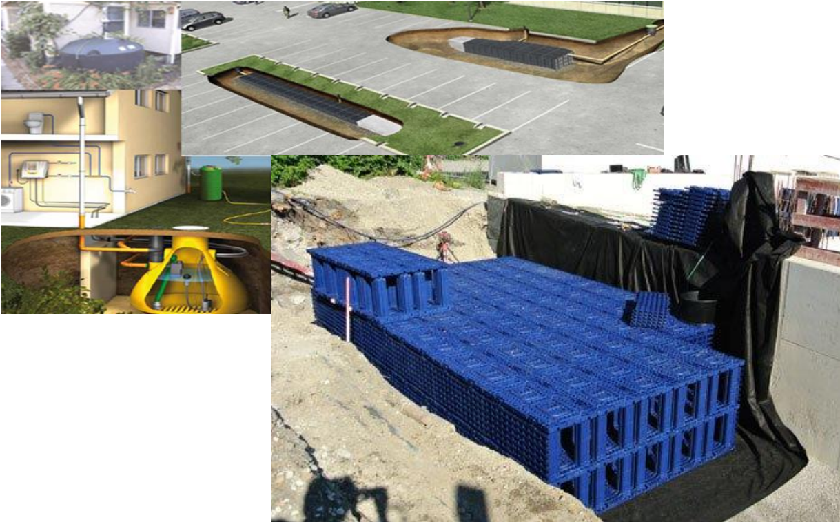
Figure 17: Underground tanks for roof rainwater retention
